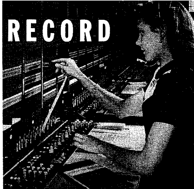
Fig. 1—A position at a No. 5 switchboard used with the A4A system for handling delayed calls.
